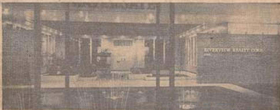
Temporary sales and exhibit building was erected in six weeks.
